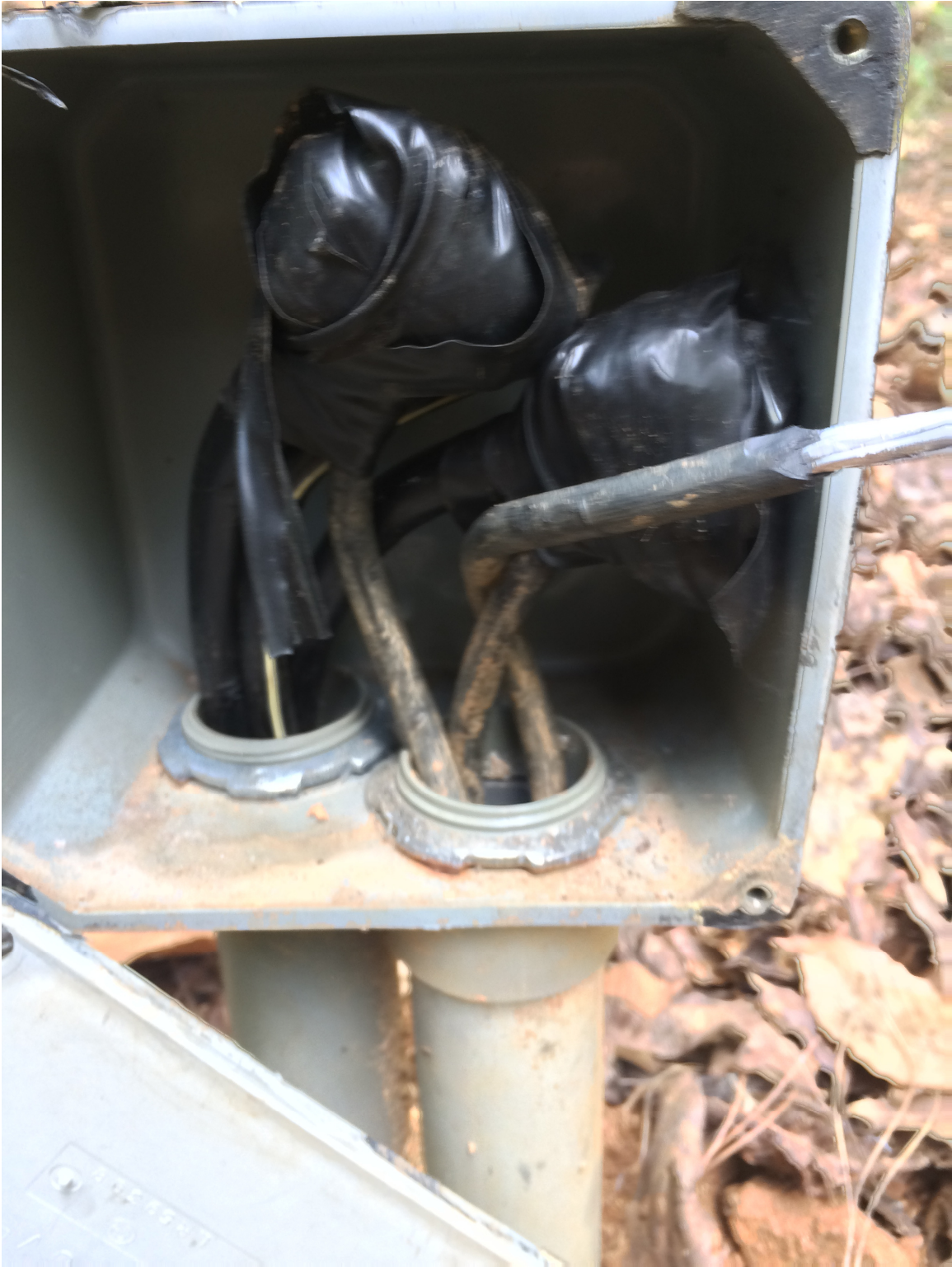
Image 2. Repair of electrical feeder.
